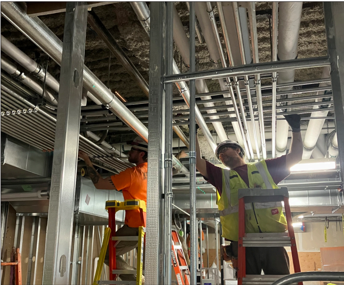
Energized Electric installing conduit at Level 2 Lewiston Phase.
