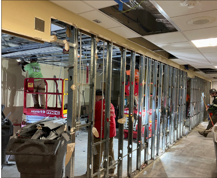
Wrecking Ball performs selective demolition in Phase 1 Palouse Phase.
