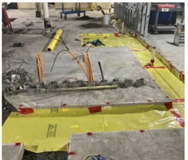
Paradise – Slab Prep
