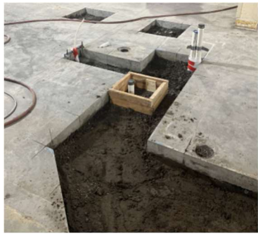
Paradise – Slab Rough-in
