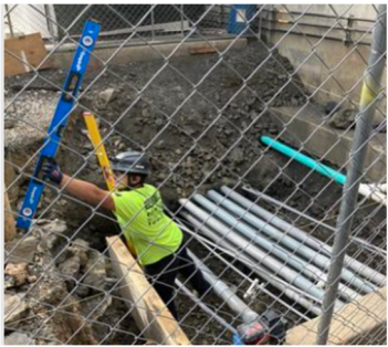
Vault Curb Prep
