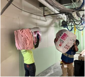
Butch – Temp Wall Insulation
