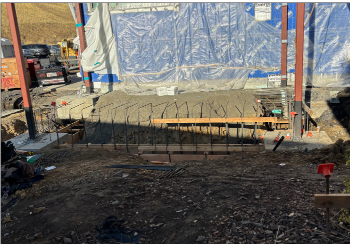
A1 PH2 Butch footing repair.
