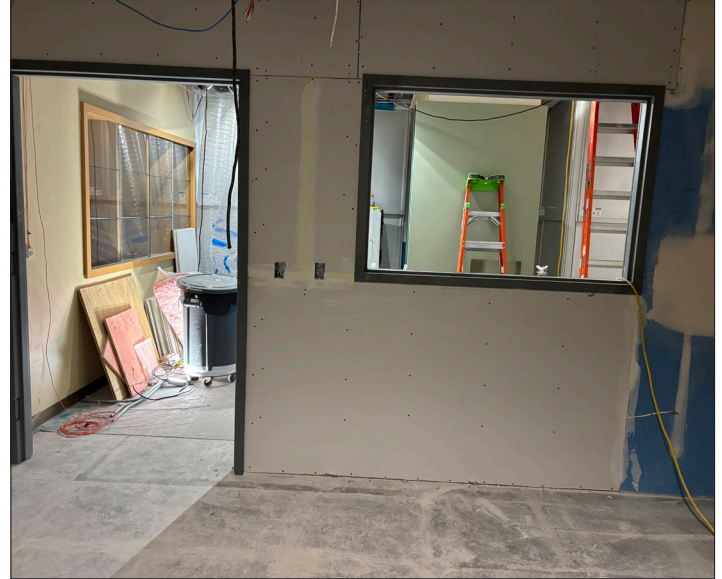
A1 North/Main progress.
